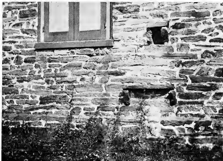
SMOKE HOLE IN WALL OF HAVERFORD MEETING HOUSE, 1700 The oldest church building in Delaware County
