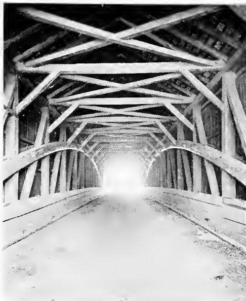
INTERIOR OF A COVERED TURNPIKE BRIDGE
