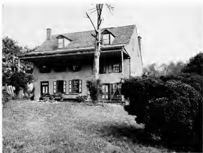
GRANGE FARM, NEAR TABOR STATION Built by Jan Luken, in 1708
