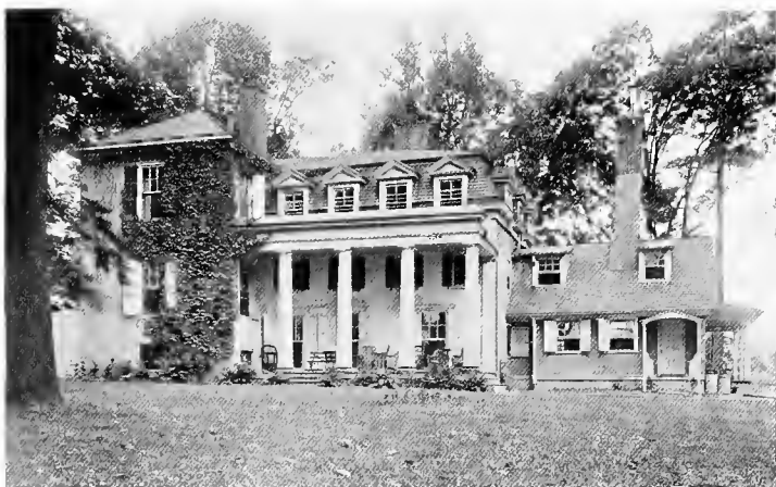
PONT READING HOUSE, ARDMORE JUNCTION
