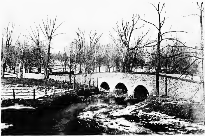
BRIDGE OVER THE POQUESSING AT TORRESDALE
