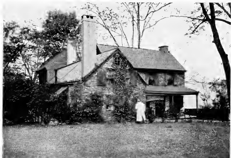
OLD FARM HOUSE Near the gate of Butler Place, the country home of Mr. Owen Wister
