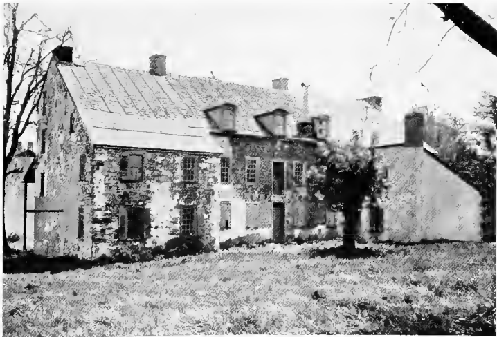
UPPER INN, REAR VIEW
