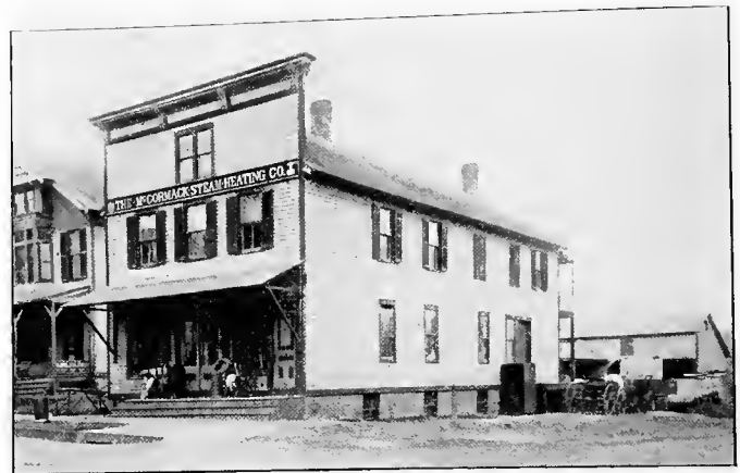
MCCORMACK STEAM HEATING CO.
