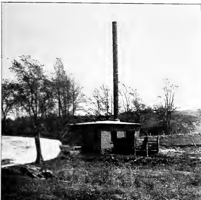
NEW PUMPING STATION.
