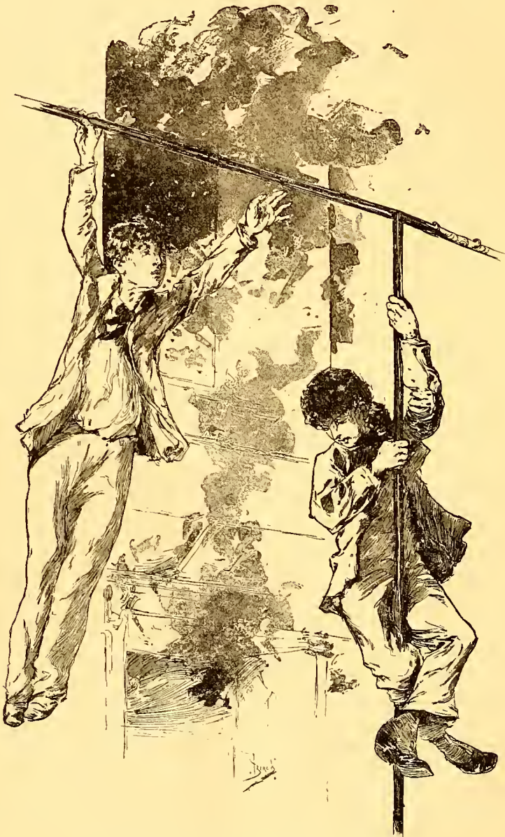
WILL AND OTIS CLIMB DOWN FROM THE BURNING BUILDING.
