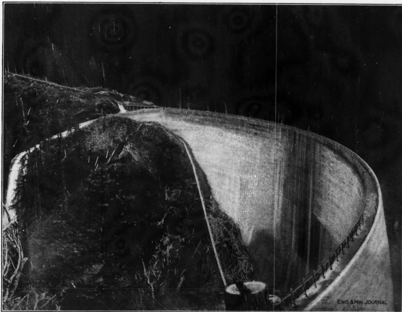
SALMON CREEK DAM OF ALASKA GOLD MINES CO. 700 ft. long and 165 ft. high.
