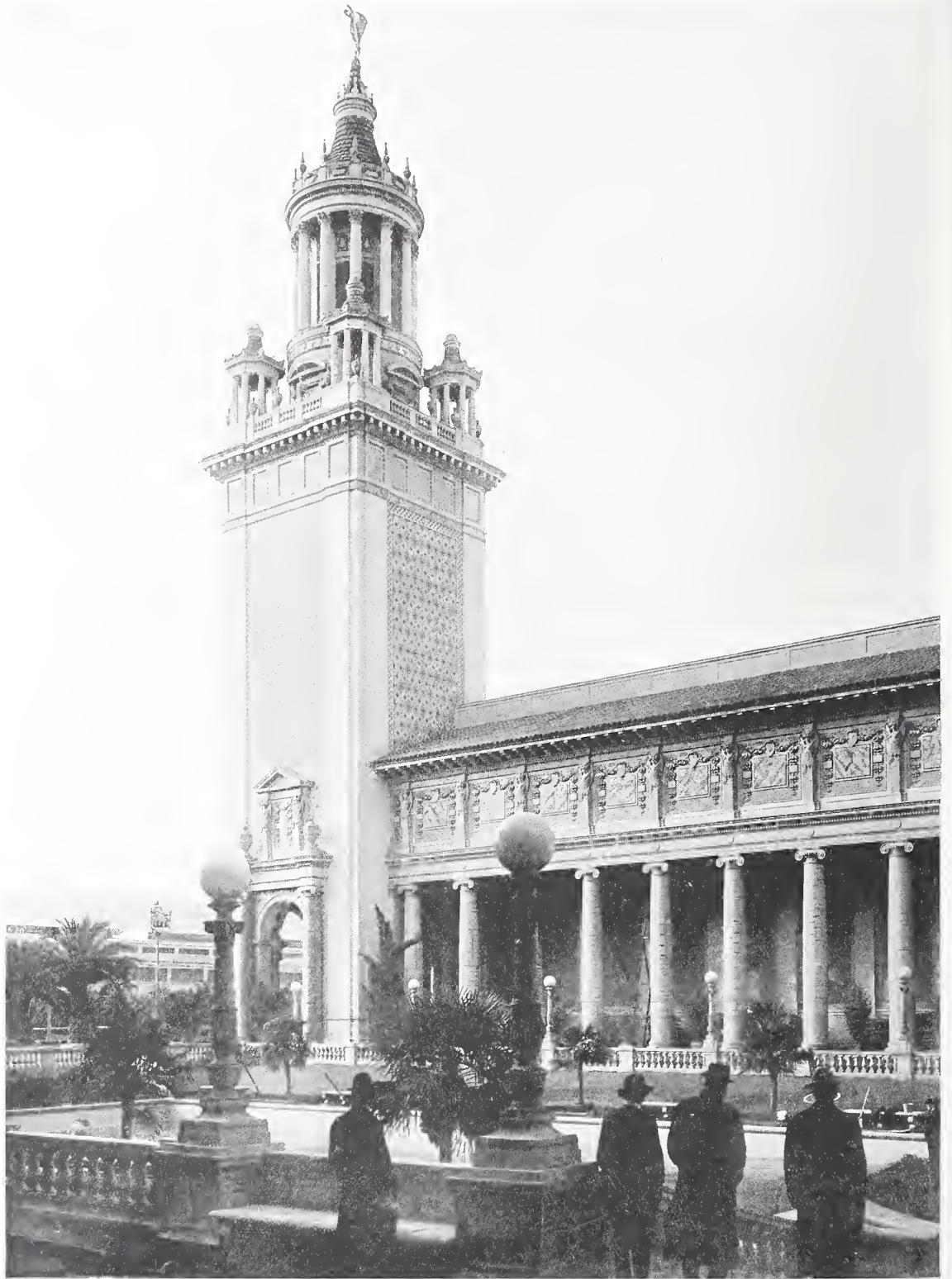
PANAMA-PACIFIC INTERNATIONAL EXPOSITION: COURT OF PALMS, SHOWING ITALIAN TOWER AND PORTION OF COLONNADE OF PALACE OF EDUCATION
