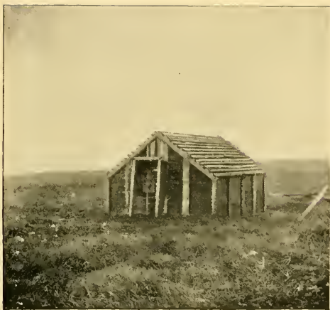
4. —WOODEN FRAME OF YURT, NORTH ROOKERY VILLAGE, BERING ISLAND.
