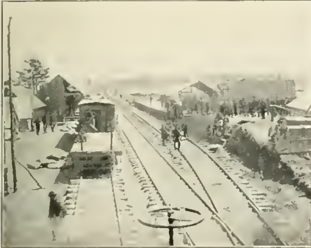
STORES AT STONEMAN'S STATION
