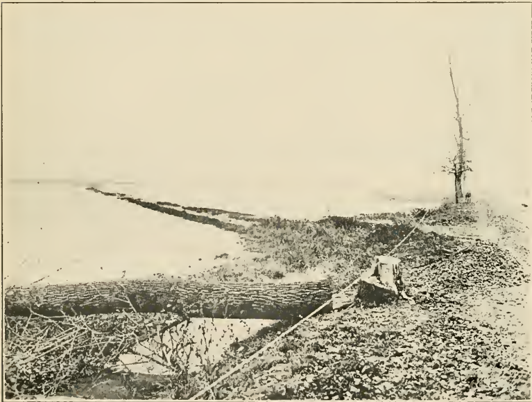
Above—German front line trenches just north of Feye-en-Haye after battle of September 12, 1918. View of wire entanglements through which 90 Division made its way.
