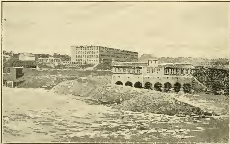
Power House, Columbia Water Power Co.
