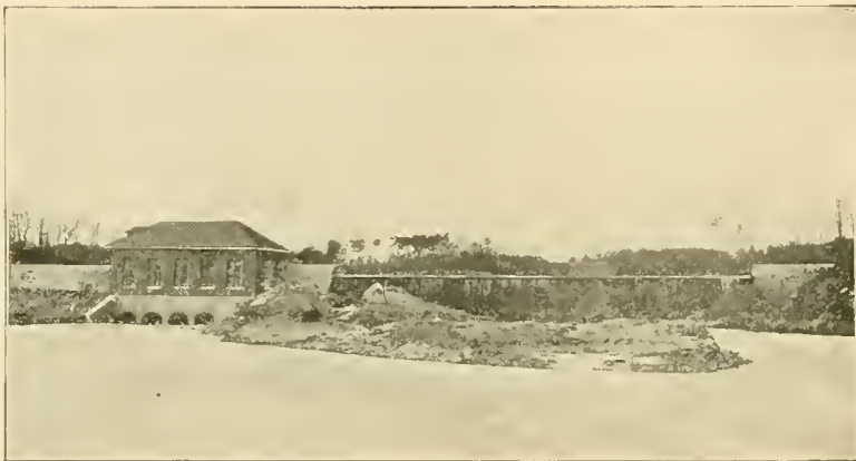
Dam and Power House, Pelzer Mfg. Co.
