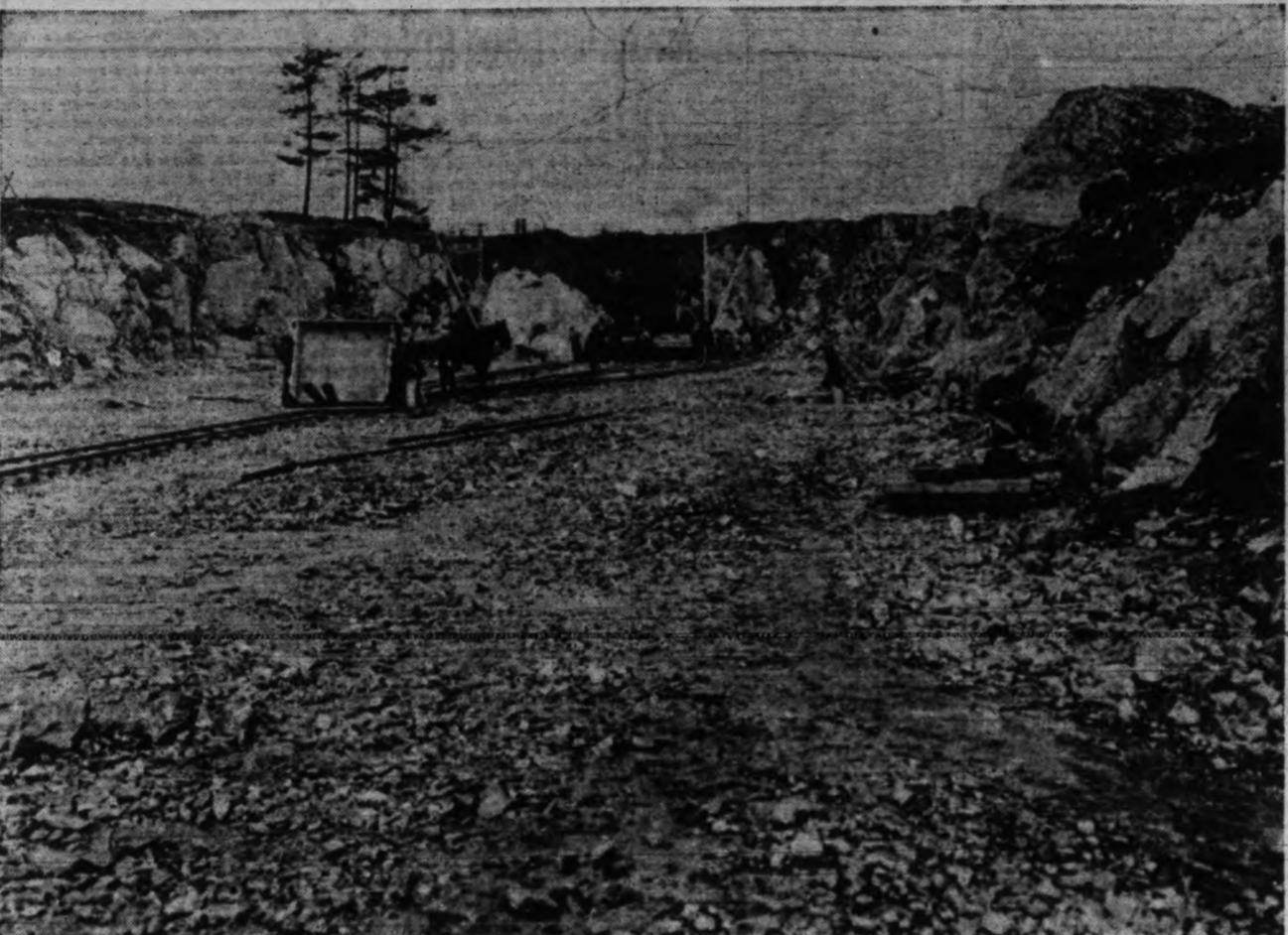
The view above depicts the rock cut in the old Indian reserve, which has been the scene of work for many months past, excavating material for the fill eastward across the swamp. The extension of Johnson street passes through a heavy knob of solid rock, which has to be opened to give access to the B. & N. Railway shops, and eventually through to Lime street, and the Esquimaux road. The noise of the explosions has served many times to remind citizens of cannonading experience. The work has been in progress under the provincial department of public works for a long period.
