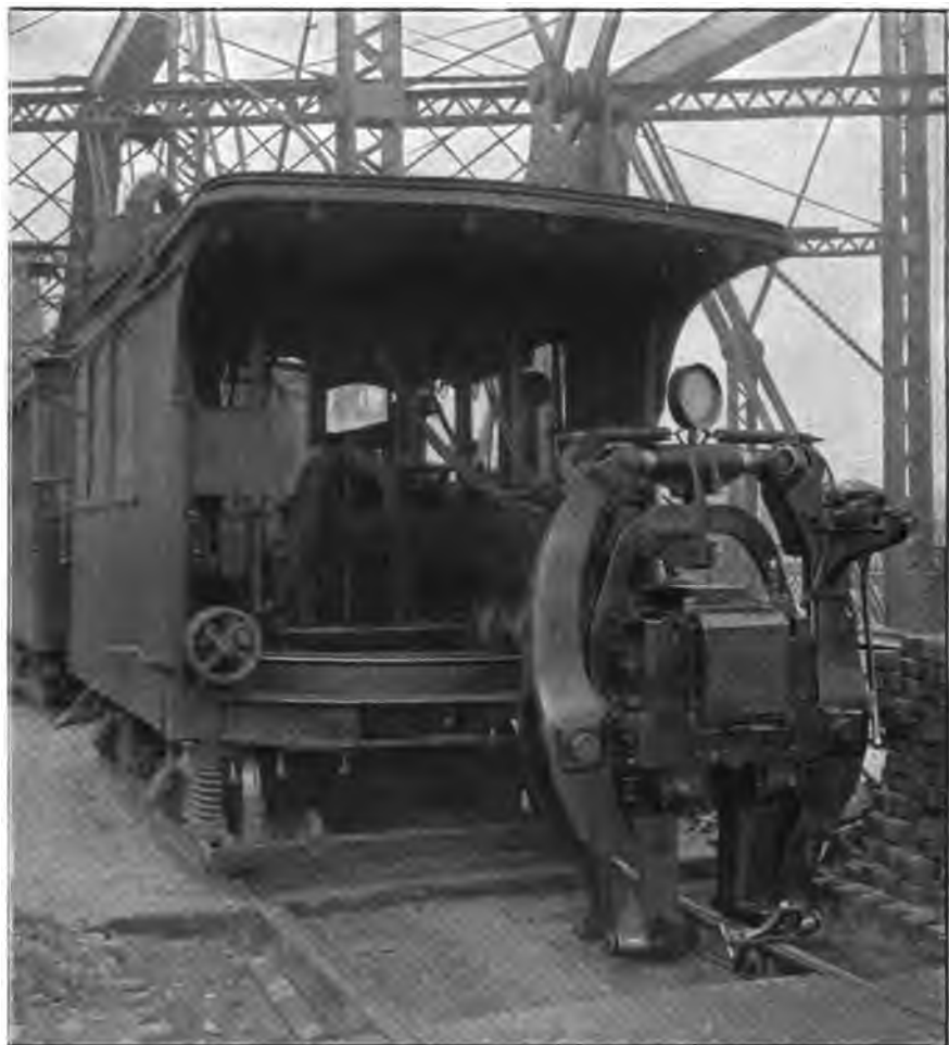
ELECTRIC RAIL WELDING ON STREET RAILWAYS, AS PRACTICED BY THE LORAIN STEEL COMPANY, JOHNSTOWN, PA., AND LONDON.
