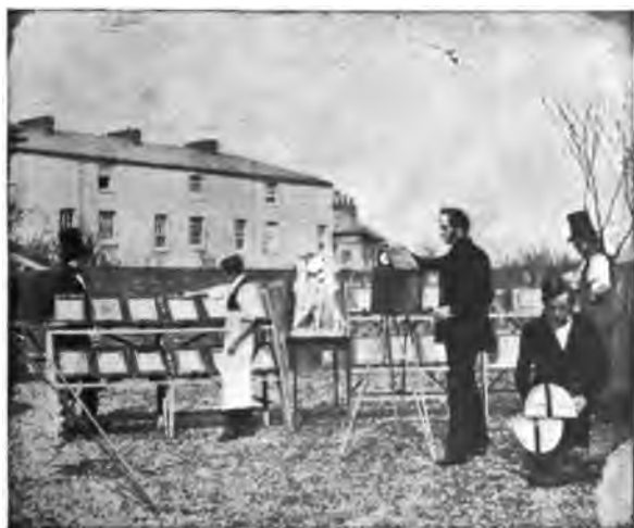
FIG. 2.—CALOTYPE PRINTING OUTFIT. From "Photominiature."
