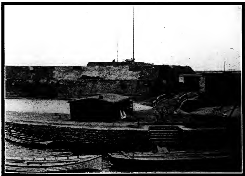
TAKU FORTS, INSIDE VIEW
