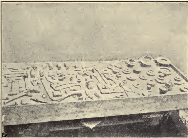
FIG. 11.—Samples of lead-castings or proofs from drop-forging dies for testing accuracy of outline.
