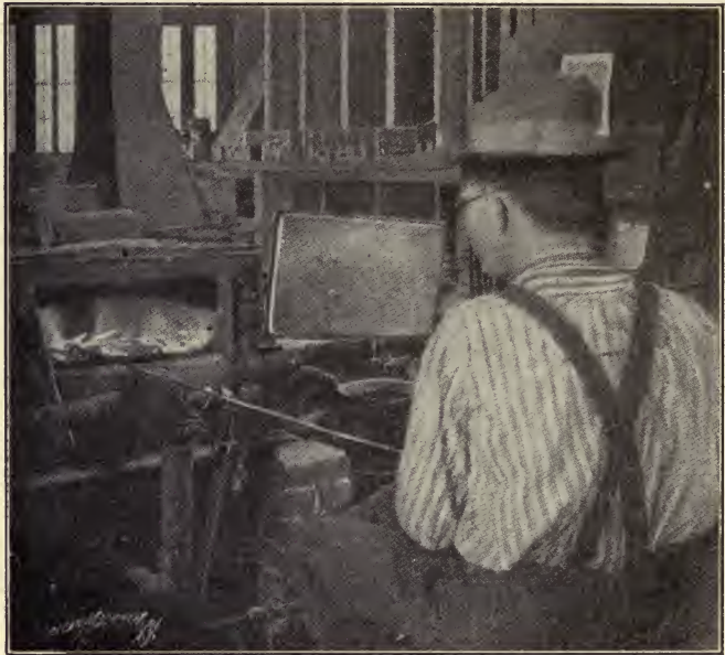
FIG. 205.—Heating flanges in muffle, using natural gas.
