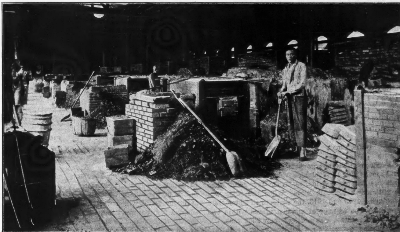
REVERBERATORY FURNACES OF WAH CHANG MINING AND SMELTING CO., CHANGSHA, CHINA
