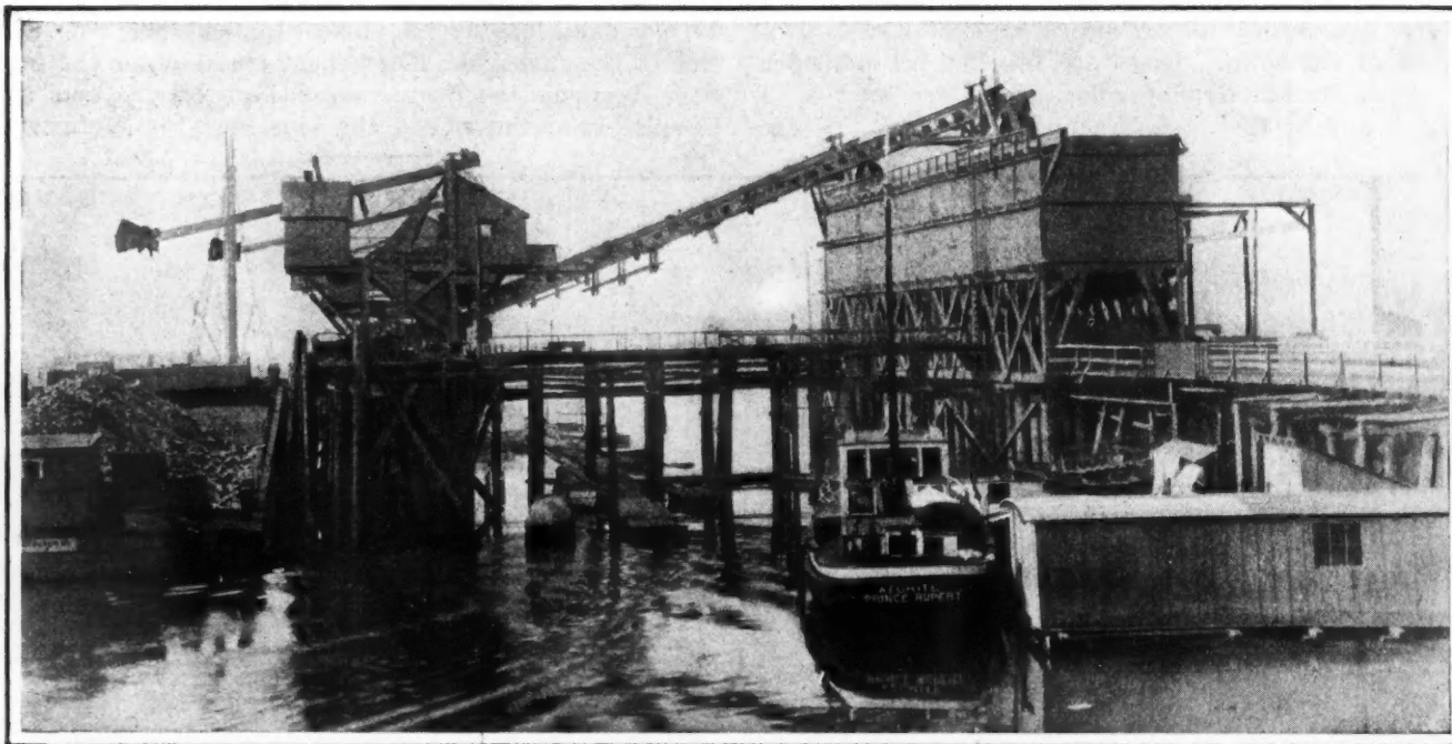
RECEIVING BINS AT ANYOX AND MEANS FOR UNLOADING OUTSIDE ORES AND FLUXES
