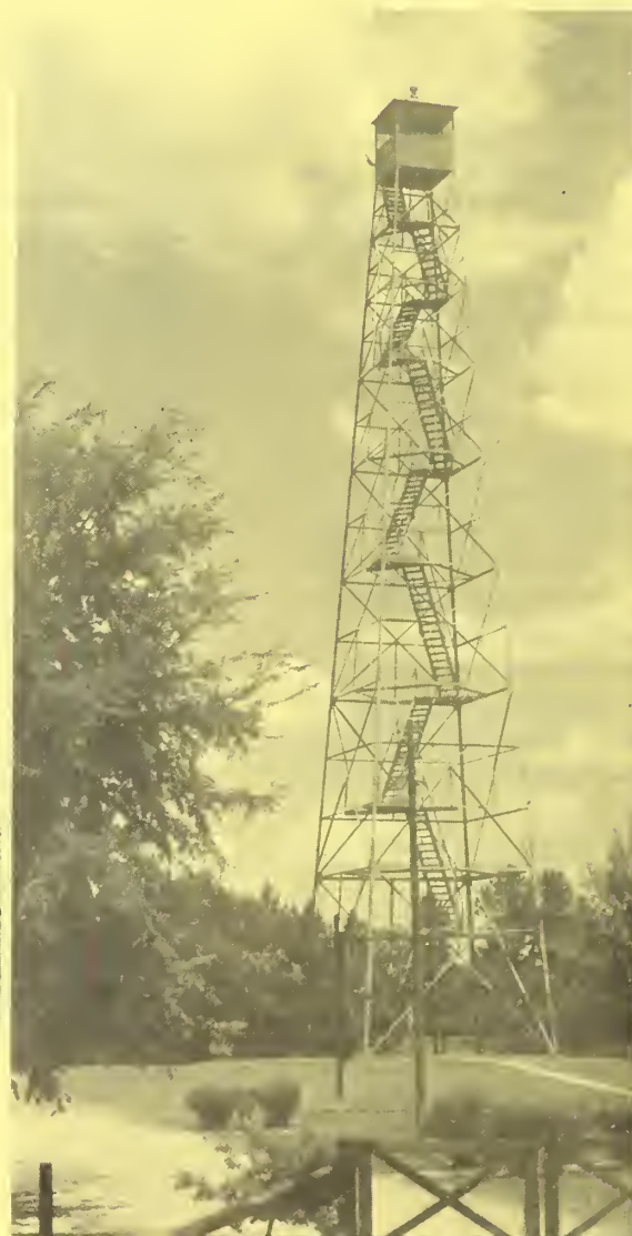
Advancements in fire detection facilities point to progress in forest fire protection that was stimulated by cooperative features of the Weeks Law.
