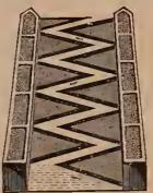
The Fish-way is constructed in the bottom of a rute of any desired width, by means of timbers rming triangles, making as signag course, hreaking he force of the water in its descent, coabling any ind of fish to ascend it. It may be constructed in a se or grade of nue foot in ten. Its opper end exided the the pool of a dam. The water "flows with multiprim switness over a smooth bottom." It does of form any "pools or eddies."
