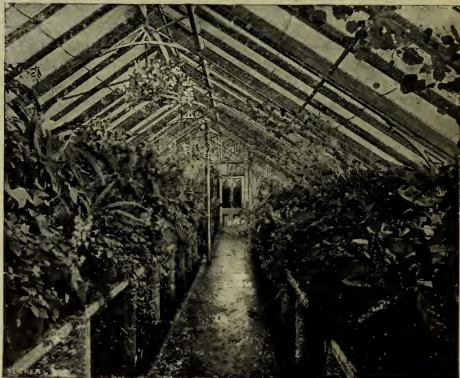
ERECTED AT NORTH FINCHLEY.
