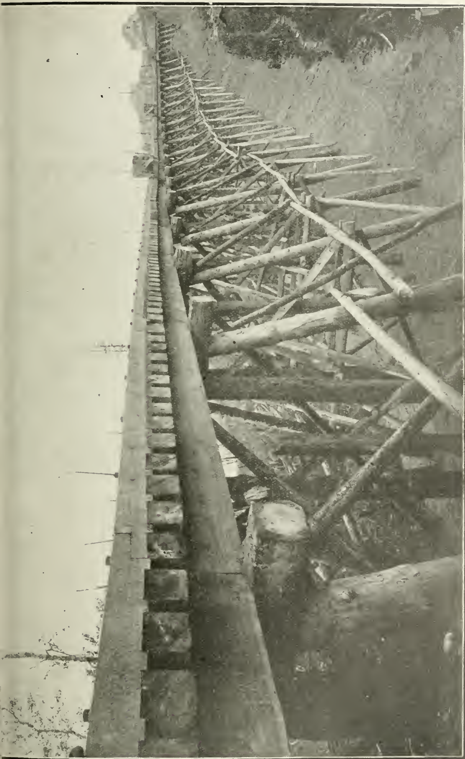
Temporary Trestle. Kerr Lake Branch.
