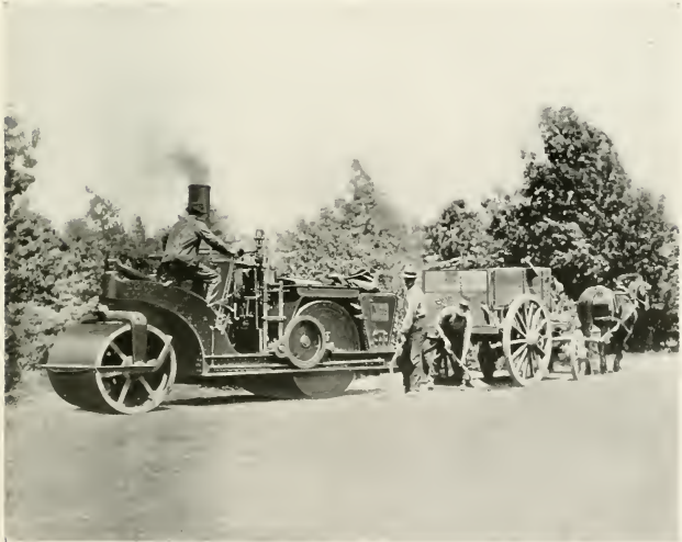
FIG. 38.—Pavement Repairs at Boston.
