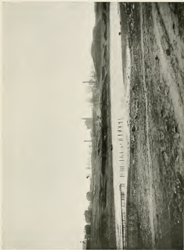
FIG. 7.—Topsoil Stripping, Piling, and Grading.
