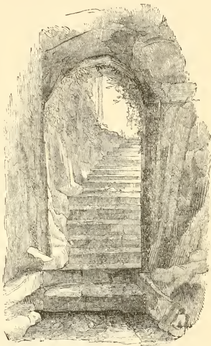
“Subterranean Passage under the Logan House.”
