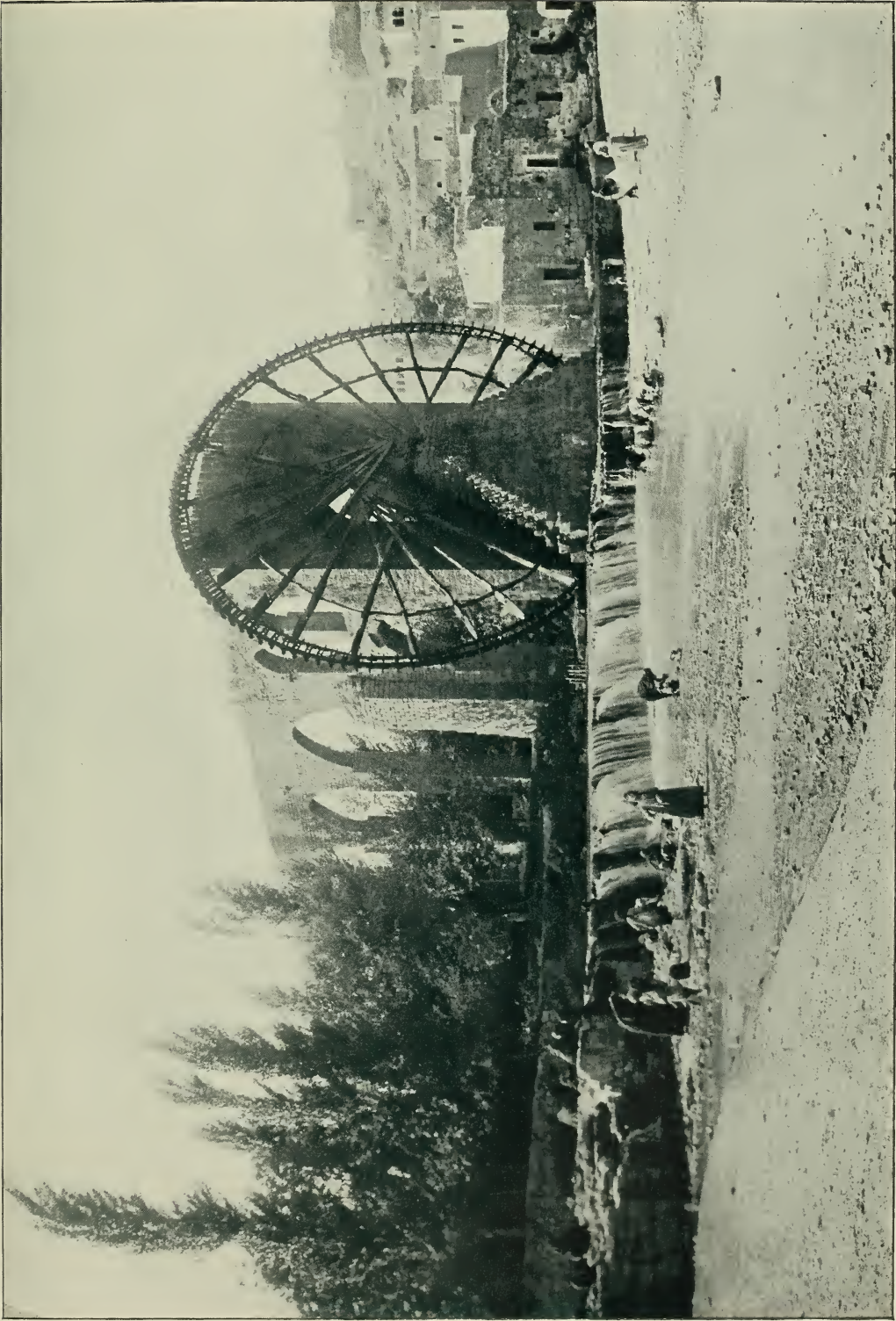
The great waterwheel at Hamâ, Syria, used for pumping the water out of the Orontes River
