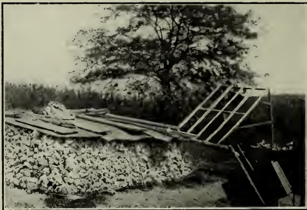
Barite "Diggings," showing windlass, rocker and stock pile of barite.
