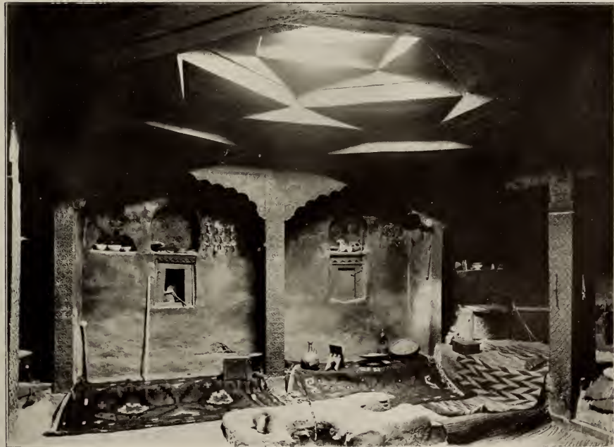
20. PARLOUR IN OBAIDULLAH'S HOUSE, MIRAGRAM. Ceiling with sky-light of characteristic construction ; below this, open fire-place ; carpets of local make.
