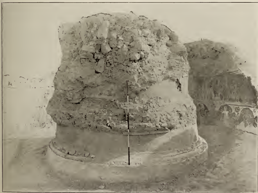
145. INTERIOR OF ROTUNDA AND STUPA IN RUINED BUDDHIST SHRINE M. V., MIRAN SITE, AFTER EXCAVATION.
