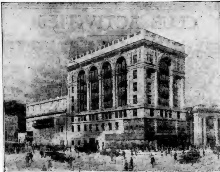
The E. F. Albee Theater, Brooklyn, N. Y., was formally opened Monday evening, January 19, as a memorial to Mr. Albee. Built at a cost of $3,000,000, it is regarded as the most modern theatrical structure in existence in point of comfort for both patron and artiste as well as its general equipment.
