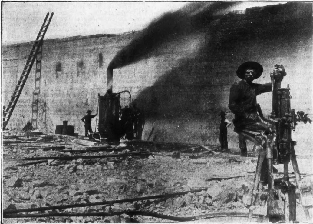
CHANNELER AND DRILL ON CHICAGO DRAINAGE CANAL.
