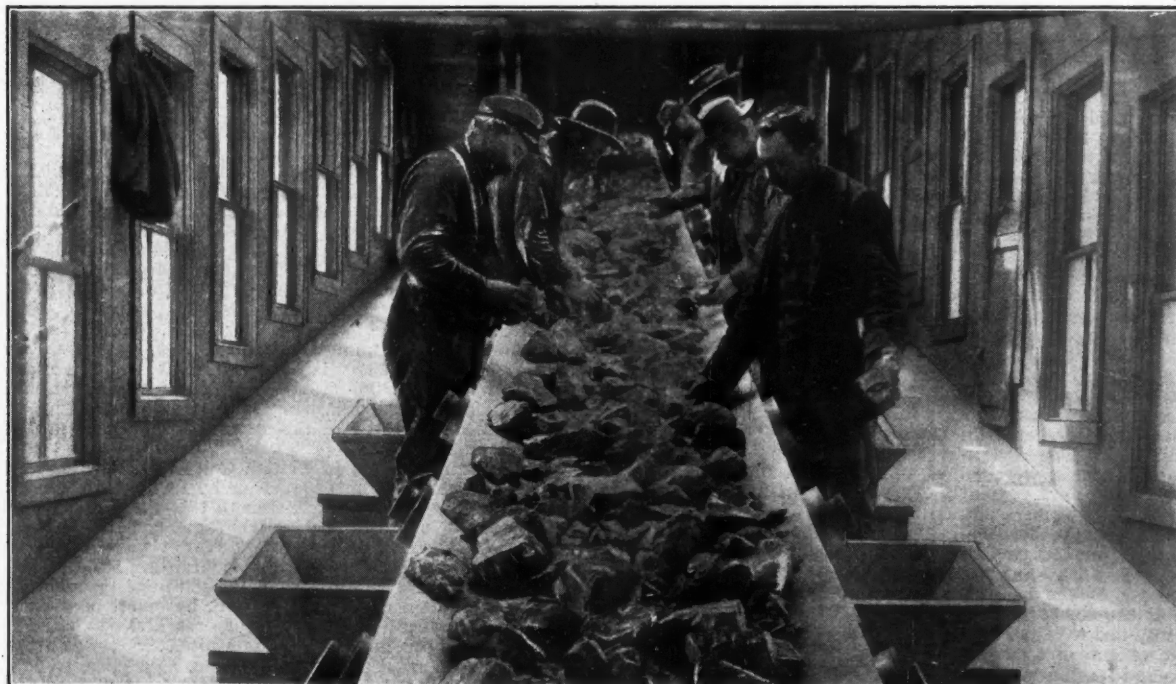
ROBINS ORE SORTING BELT, BRITISH COLUMBIA COPPER COMPANY'S WORKS.
