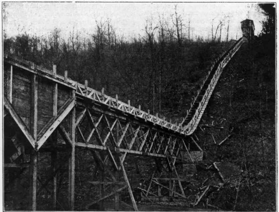
COAL CONVEYOR, URSINA COAL COMPANY, HUMBERT, PA.
