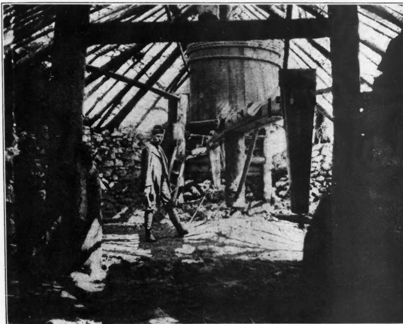
HORSE-WHIM AT VLADIMIR SHAFT, YUSPENSSKI MINE.
