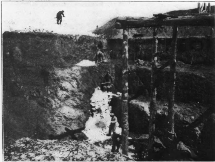
OPEN CUT AT DJAM-BHOULDI MINE.
