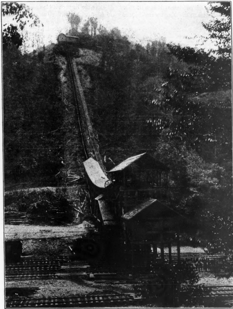
RETARDING COAL CONVEYOR AT THACKER MINES, WEST VIRGINIA.
