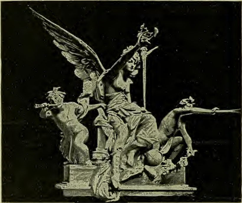
SCIENCE, ADMINISTRATION BUILDING. ( Karl Bitter. )
