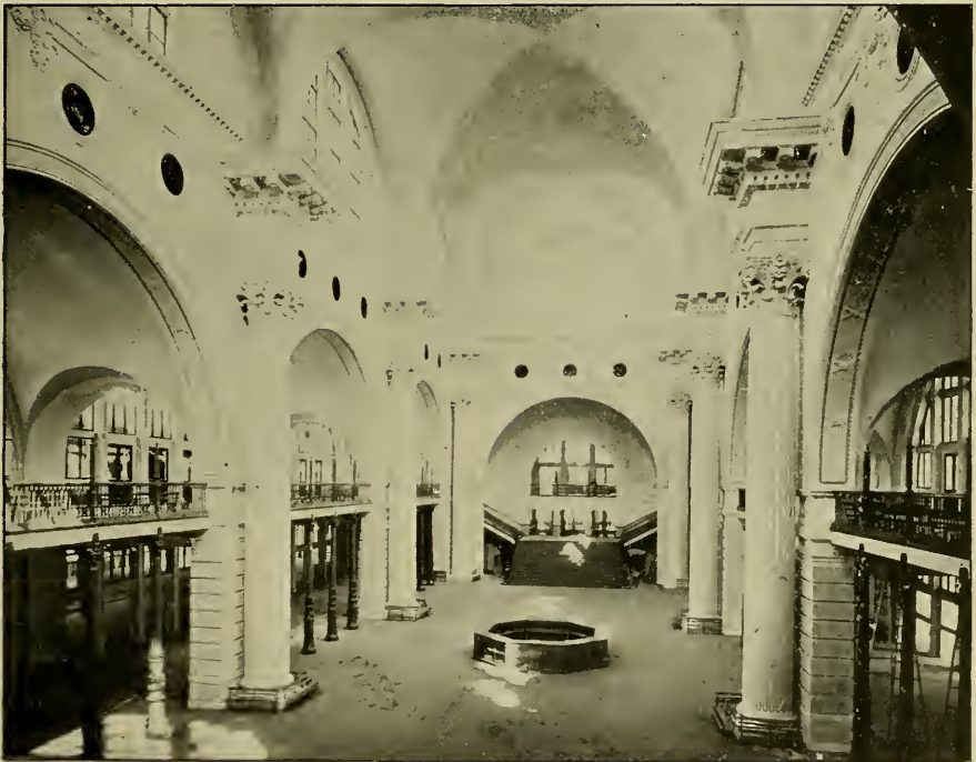
INTERIOR OF TERMINAL STATION.
