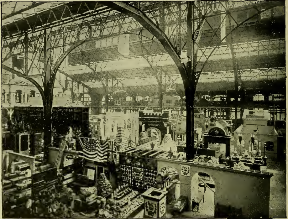
VIEW IN NORTH END OF BUILDING.
