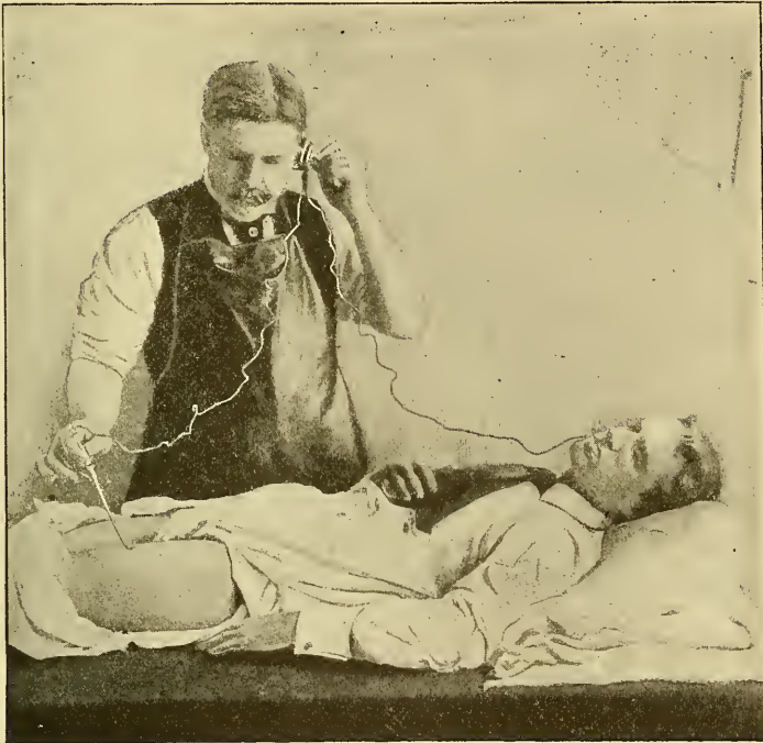
FIG. 199.—Method of Using the Telephone Bullet Probe.
