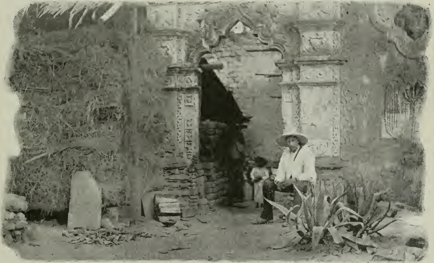
DWELLING IN A RUINED CHURCH.
