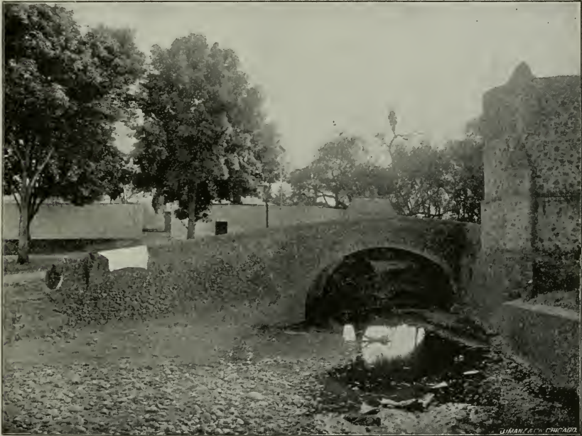
OLD BRIDGE, COYOACAN.
