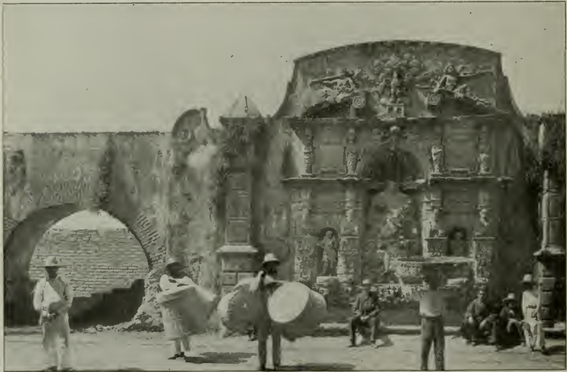
SHRINE IN THE OLD AQUEDUCT.
