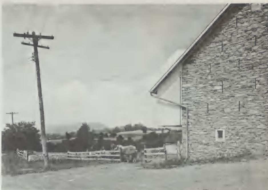
One of the big stone barns which has stood for years, notice the loopholes which ventilate the hay; these barns are a familiar part of the Pennsylvania landscape
