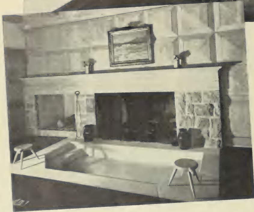
The living room, jutting out towards the tip of the peninsula, has been designed to take full advantage of the views over the lake. The fireplace detail shows the interesting "sunken hearth" treatment and the stone storage compartment for logs at the left
