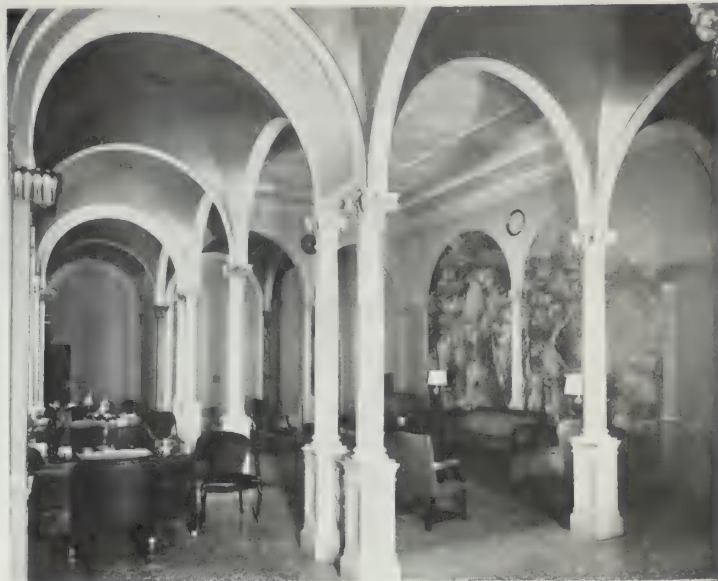
A section of the Gallery, Fifth Avenue Office
