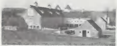
Buildings on the McCord Farm, near Philadelphia. Lightning Protective Installation by Hazard
