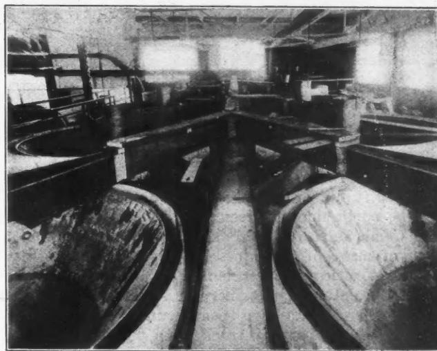
Settling cones in classification section
