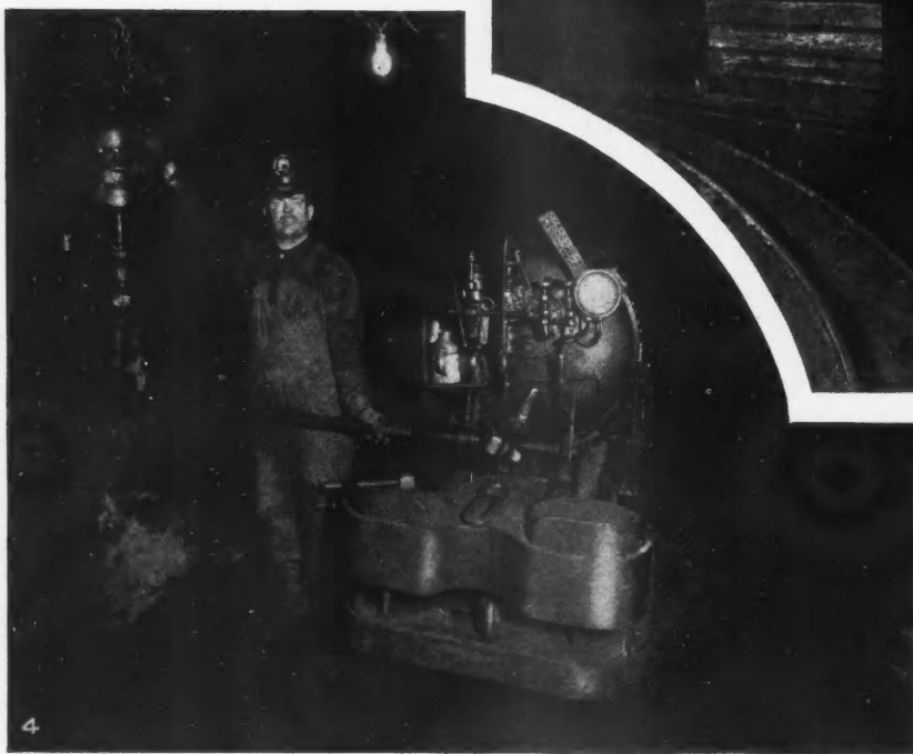
3—Ventilating fan used underground. 4—Charging a compressed-air locomotive underground.
