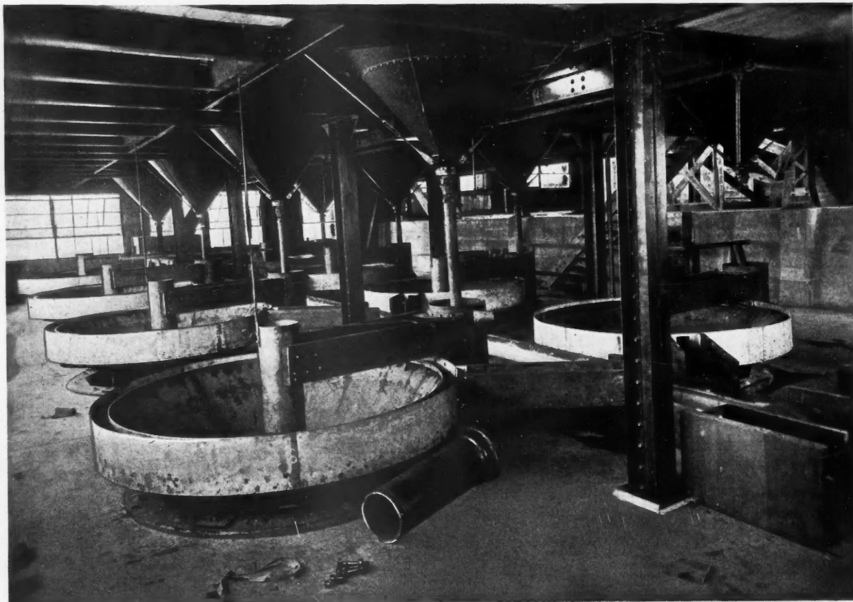
Settling cones in classifying section of mill
