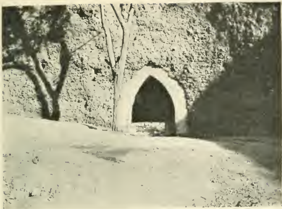
A Moorish Well near the Sacro-Monte
