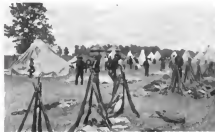
ON THE MARLBOROUGH TRENCH FOR THE NIGHT
