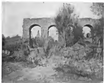
REMAINS OF THE OLD ROMAN AQUEDUCT.
