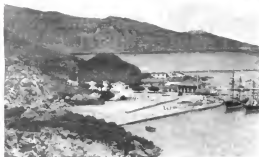
TAIKUN, ONE OF THE NORTHERN TREATY PORTS
