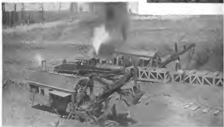
STRIPPING AND MINING SIDE BY SIDE
