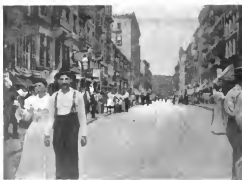
HIGGE STREET, LOOKING NORTH FROM BOWLING STREET
