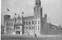
CENTRAL ARMORY FOR THE CLEVELAND NATIONAL GUARD
