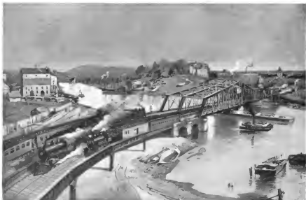
IMPROVED RAILWAY ENTRANCE TO MANHATTAN ISLAND, NOW UNDER CONSTRUCTION, SHOWING THE NEW STEEL DRAWBRIDGE OVER THE HARLEM RIVER SHIP CANAL AND THE VIADUCT APPROACHES—DRAWN BY W. LEWIS SCOTT, JUN.
