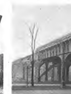
CROSSING ARLAND BOULEVARD, LOOKING WEST.
