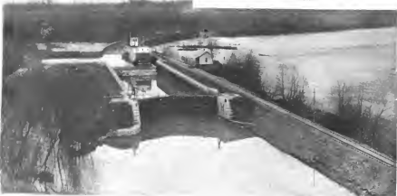
LOCK NO. 1 AND AQUEDUCT.
