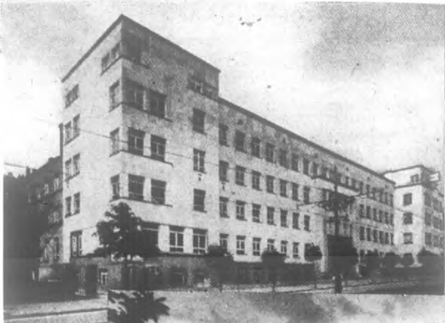
The Ministry of the Interior at Sofia, a fine specimen of modern architecture.
