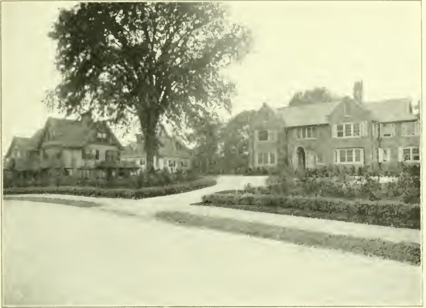
Homes on Burnham Road, Newton.
