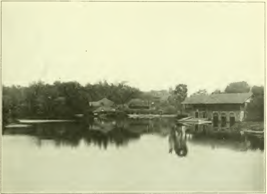
A View from Weston Bridge, over the Charles, at Riverside.
