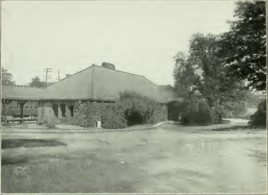
The Station, in its Garden-like Grounds, at Auburndale.
