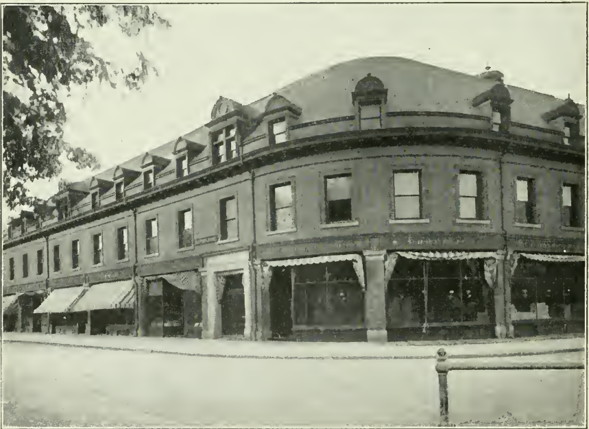
Bray's Block, with its Stores and Offices at Newton Centre.
