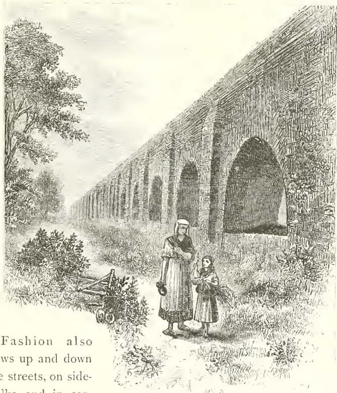
SAN COSME AQUEDUCT, CITY OF MEXICO.
