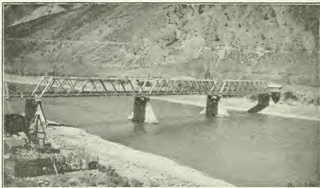
Thompson River at Spences Bridge. (Metering Station.)
