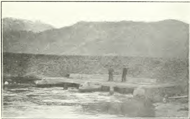
Reclamation—Pitt Meadows Dyke and Sluice Gates.
