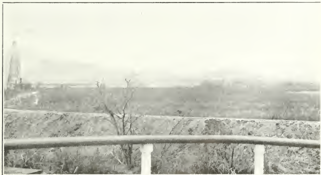
Reclamation-Pitt Meadows Pump House and Sluice Gates.
