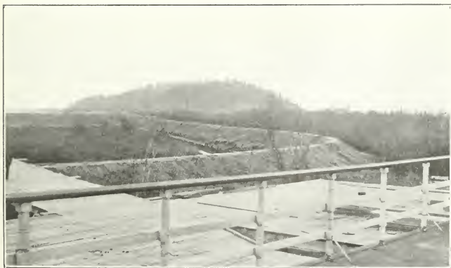
Reclamation-Pitt Meadows Dyke South of Sturgeon Slough.
