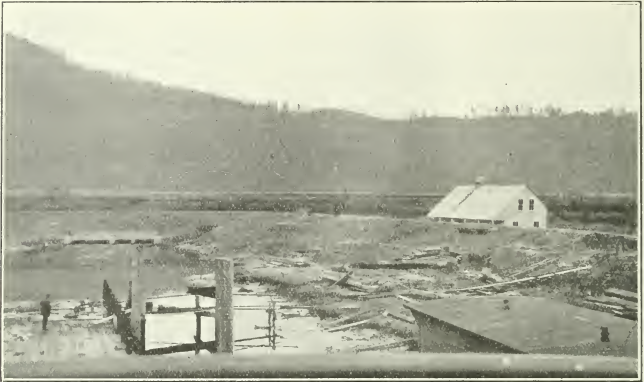
Reclamation-Pitt Meadows Dyke South of Sturgeon Slough.
