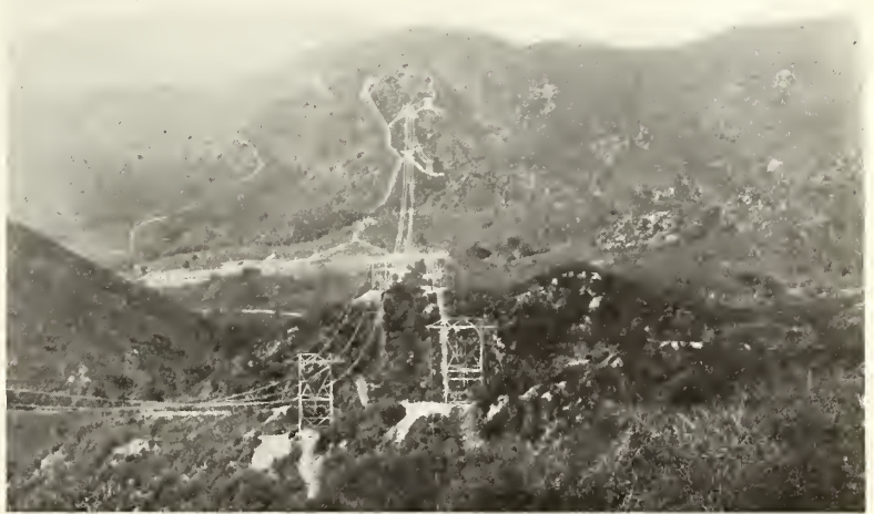
THE TRANSMISSION LINES THAT CARRY THE CURRENT OVER THE MOUNTAINS.
