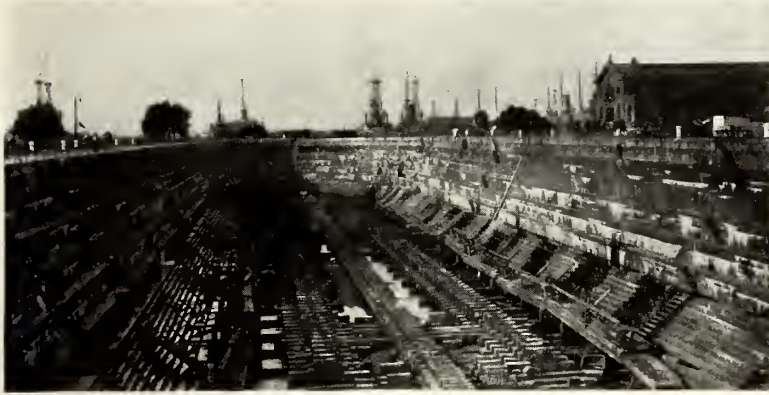
A CONCRETE DRY-DOCK 750 FEET LONG.
