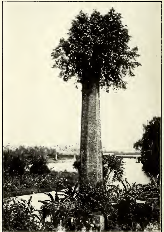
A TREE GROWING OUT OF THE TOP OF A CHIMNEY.
