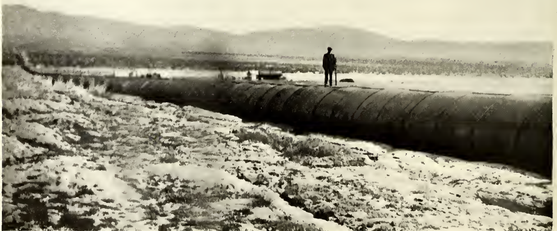
THE COLLAPSED ANTELOPE VALLEY SIPHON RETURNING TO SHAPE AFTER THE WATER WAS TURNED IN.
