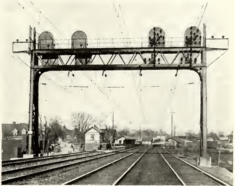
THE NEW BLOCK-SIGNAL BRIDGE.
