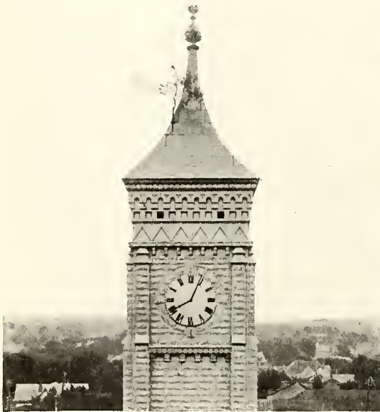
A NEARER VIEW OF THE TREE ON THE TOWER.
