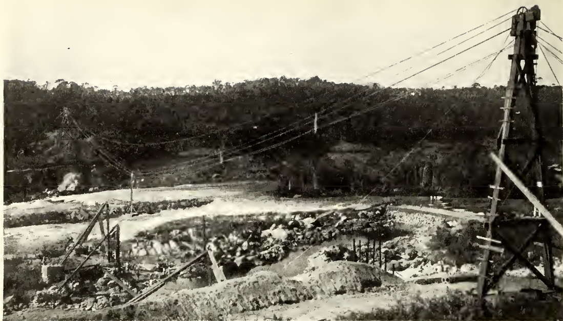
THE CABLEWAY ON THE RIO PINTO.
