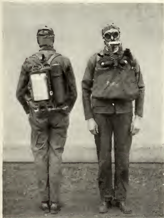
TYPES OF ARTIFICIAL BREATHING APPARATUS WORN BY BUREAU OF MINES RESCUERS AT COAL-MINE EXPLOSIONS.
