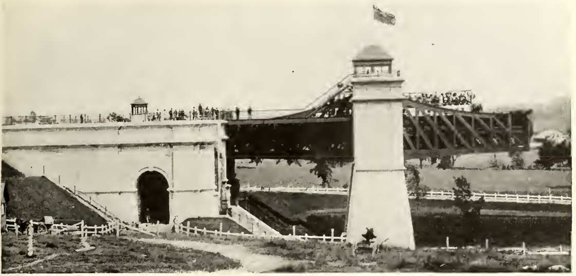
A CANAL-BOAT IN THE LOCK-LIFT AT THE UPPER LEVEL.
