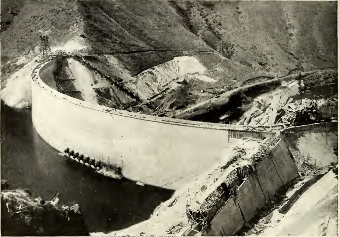
THE UPSTREAM SIDE OF THE GREAT ARROWROCK DAM ON THE BOISÉ RIVER, IDAHO.
