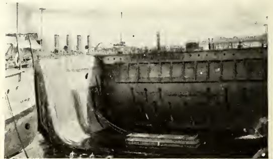
THE CAISSON THAT CLOSES THE ENTRANCE OF THE DRY-DOCK.
