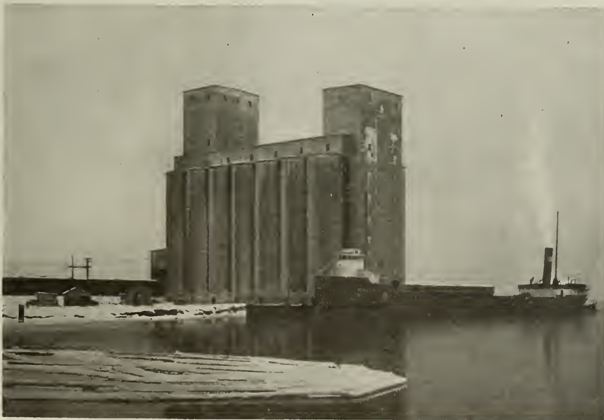
NEW TRANSFER ELEVATOR AT OWEN SOUND, ONT., CANADA
