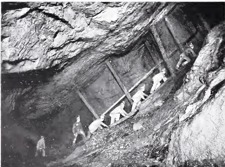
Miners climbing to the Surface from a Cornish Tin Mine.
