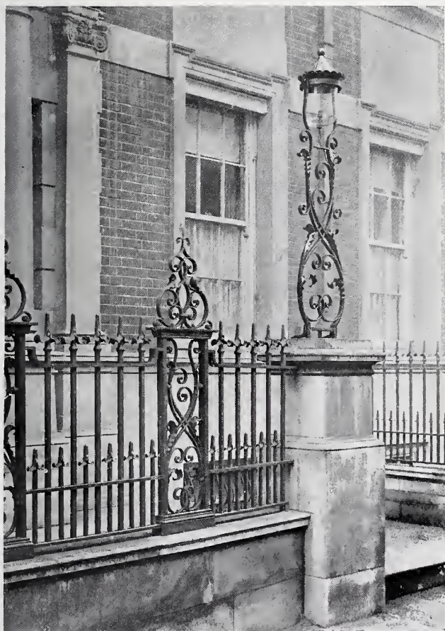
Forged Iron Railing and Standard at 32, Green Street, Park Lane for the Rt. Hon. Lord Ribblesdale.
