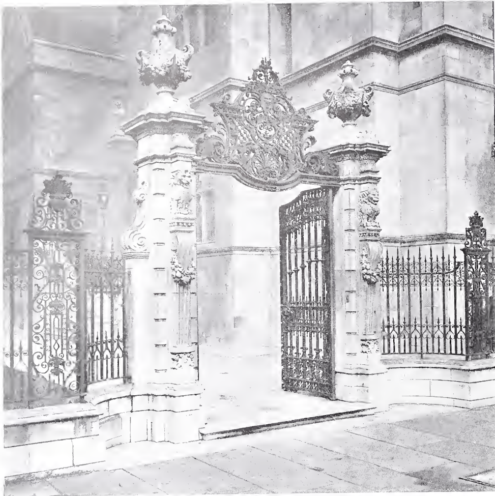
Gates, Railings and Grille at the Astor Estate Office, Victoria Embankment, for W. Waldorf Astor, Esq.
