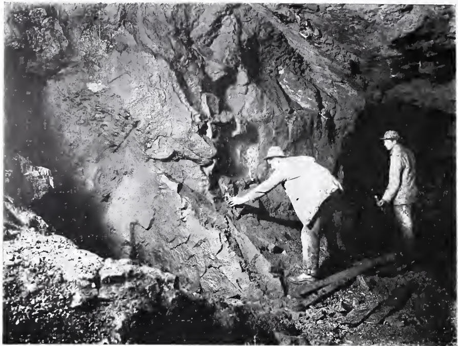
Two Holes charged ready for blasting in King Edward Mine, Cornwall.
