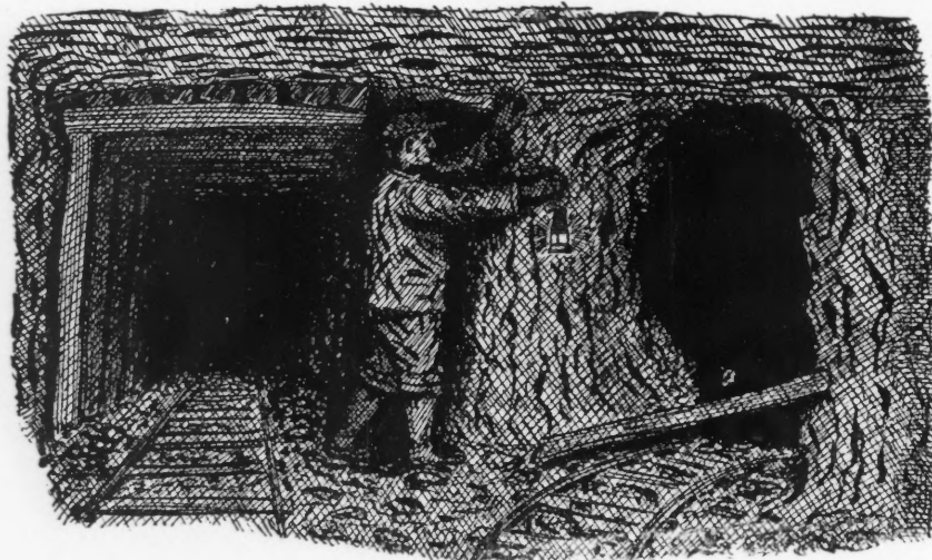
FIG. 1 CLOSING A DANGEROUS ROOM.
