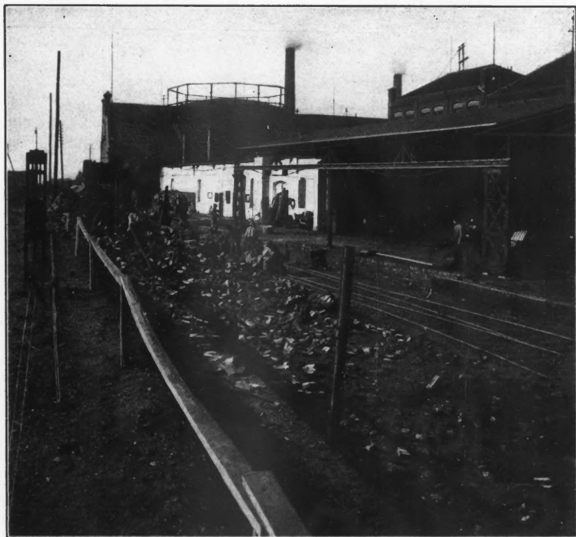
FIG. 4. THE CHIMNEY FELLED.
