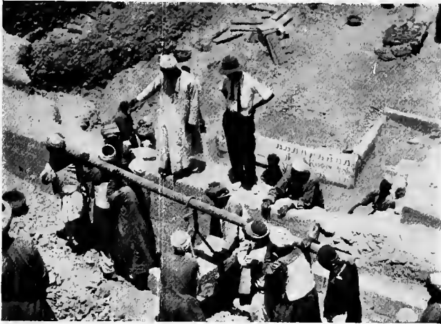
FIG. 23. METHOD OF CARRYING BLOCKS
