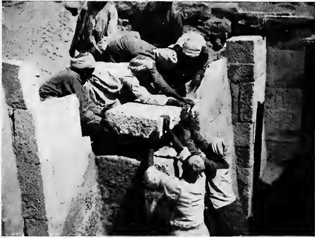
FIG. 20. REMOVING BLOCKS FROM FAÇADE
