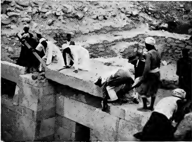
FIG. 16. REMOVING LINTEL OF MAIN DOORWAY
