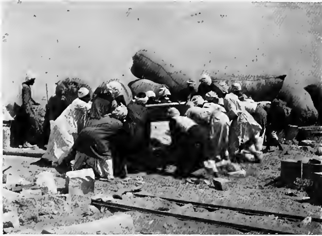
FIG. 18. PACKING LINTEL OF MAIN DOORWAY
