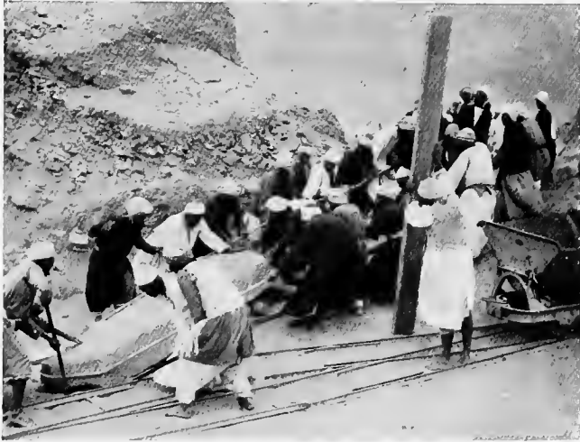
FIG. 17. HAULING LINTEL OF MAIN DOORWAY
