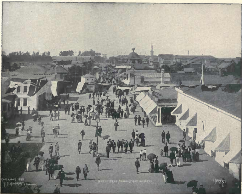
NORTH FROM ADMINISTRATION ARCH.
