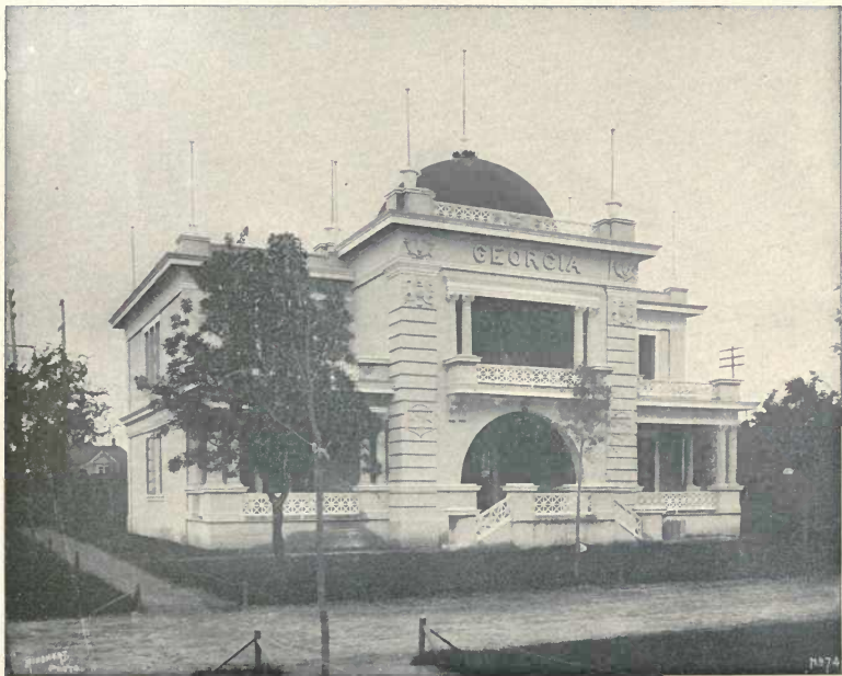
GEORGIA STATE BUILDING.
