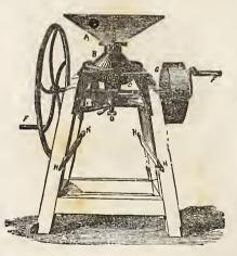
HAND AND FOWER GRAIN MILLS—Adapted for grinding grain, coffec, or spices, as may be desired. They grind from one to two bushels per hour, but can be so constructed as to run by other power, giving, of course, a proportionably increased amount of flour or meal per hour.
