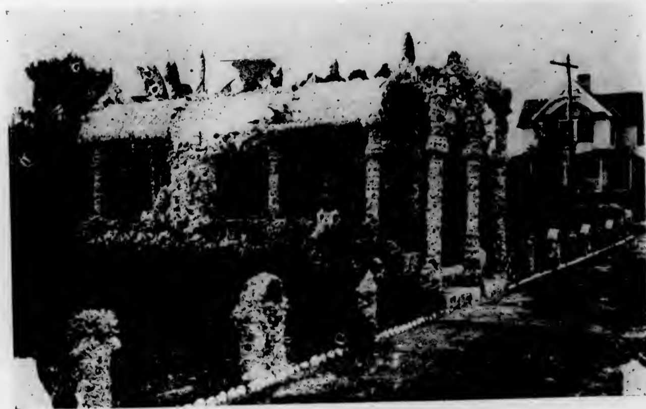
Shell House and Fence built of sea-shells by Owen Albright (He can be seen sitting in doorway) Courtesy St. Petersburg Board of Trade
