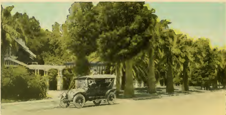
Palms in a residence street.
