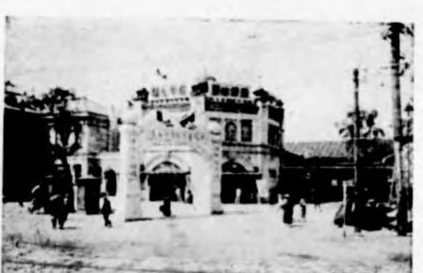
Namba Station, Osaka 場車停渡難阪大
