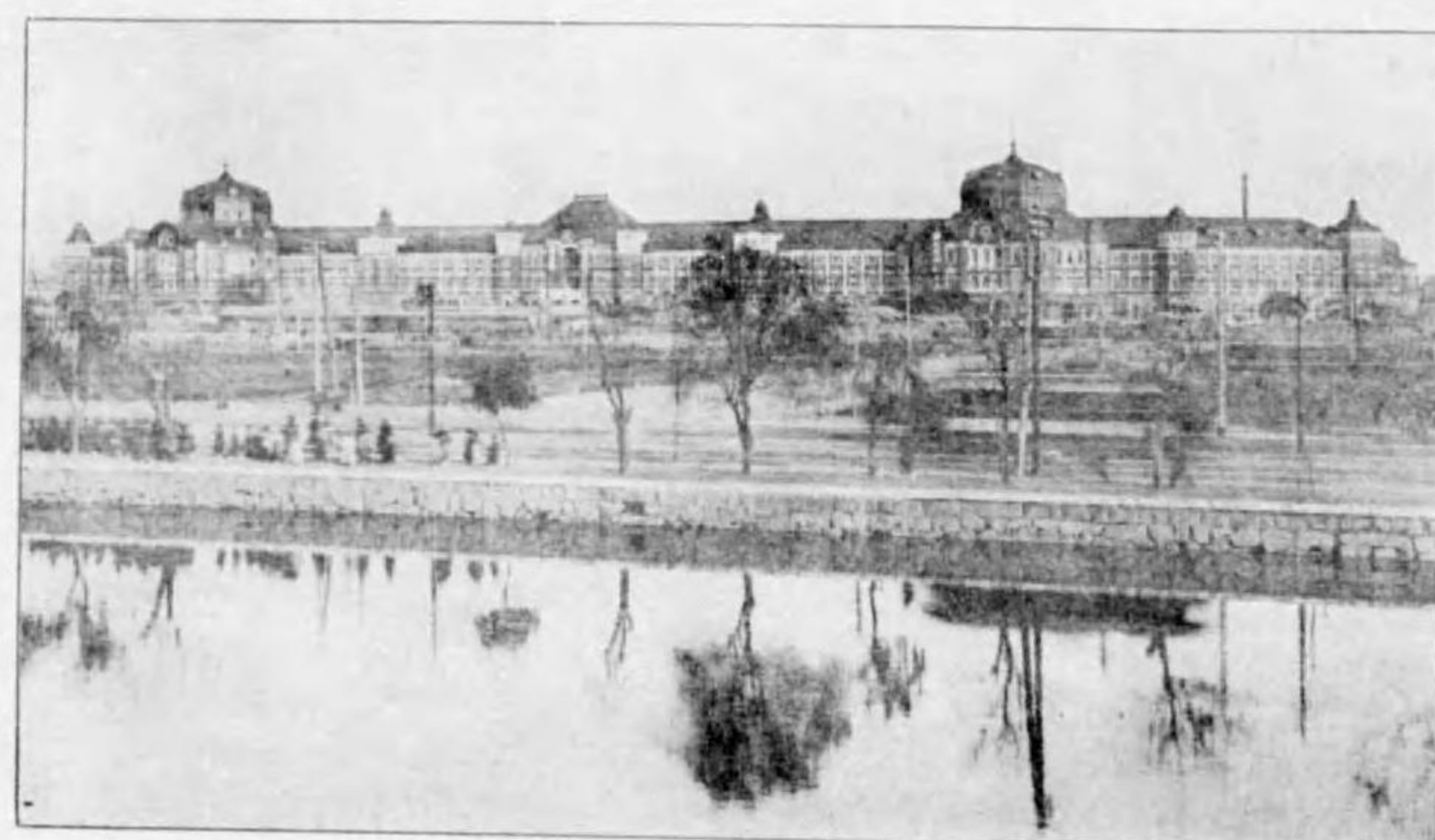
Central Station 場車停央中
