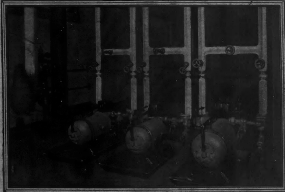
CRANETILT NON-RETURN STEAM TRAPS IN THE CALUMET PLANT OF THE COMMONWEALTH-EDISON COMPANY, CHICAGO
