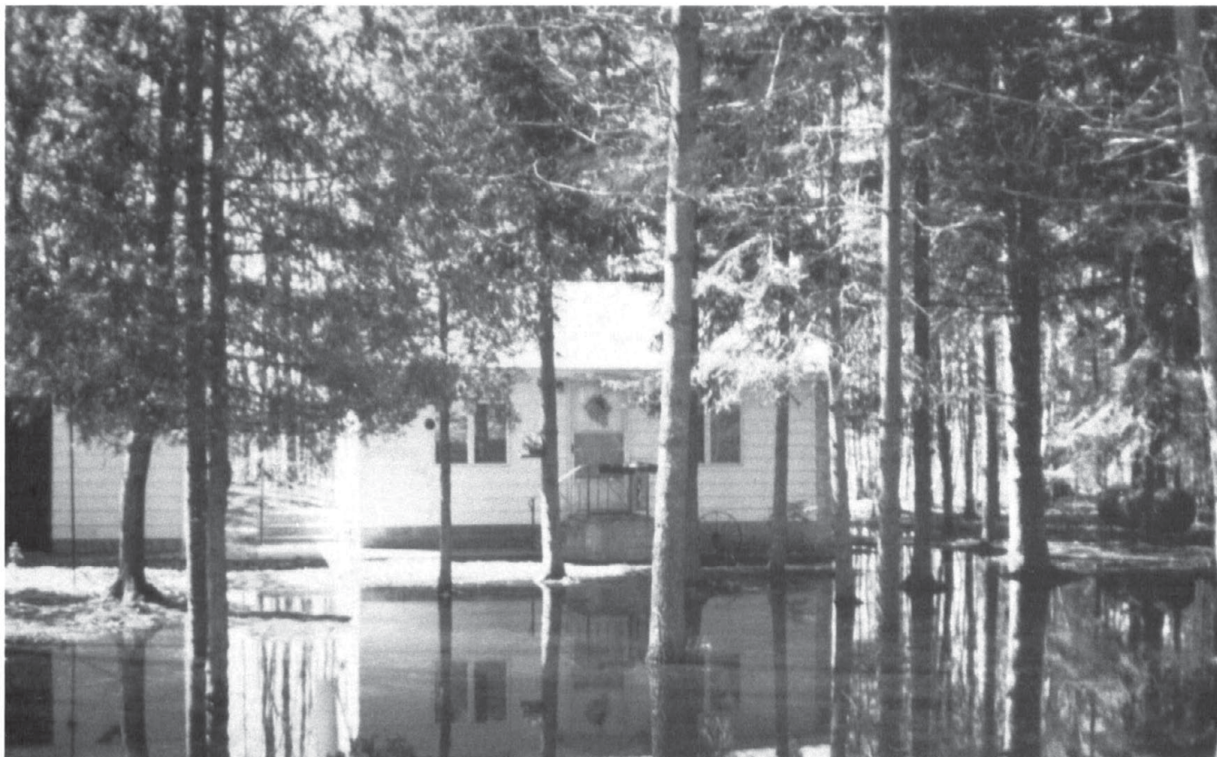
Figure 8.—Areas of Tawas-Au Gres complex, 0 to 4 percent slopes, are near Lake Huron and are seemingly attractive building sites, but ponding in the lower areas is a common problem.
